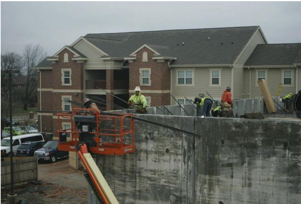
A construction worker uses a lift to raise 20-foot rods of rebar to the roof Wednesday, March 18, 2015, as a crew lays the steel reinforcing to complete a concrete storm shelter at OU Traditions Square West apartments in Norman.
